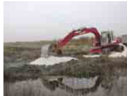
Constructing the outflow gravel filter
