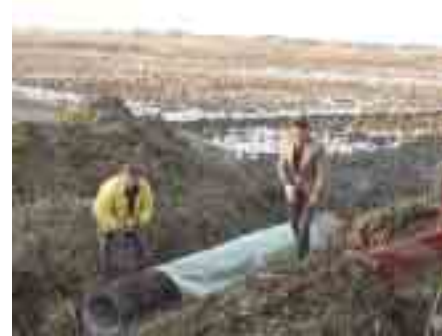
Installing Pipes for the inflow into the filter
