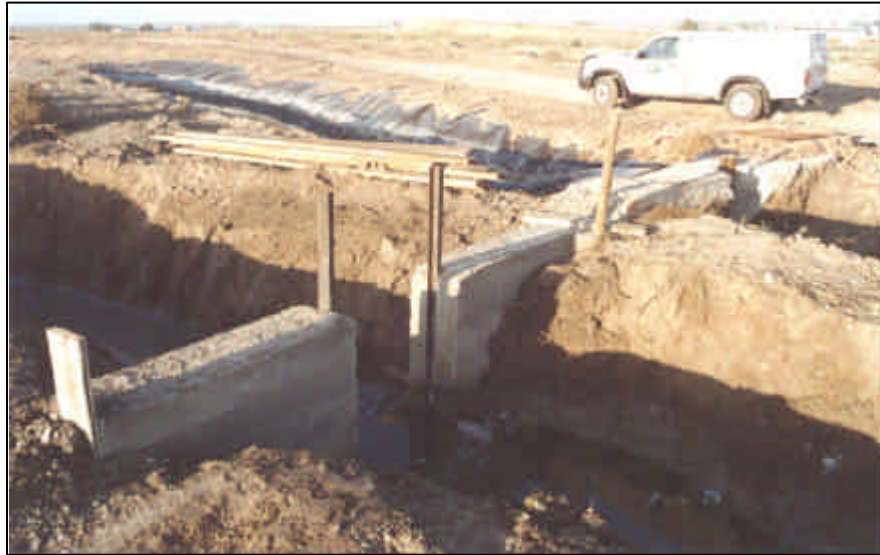
Floodgates under construction
