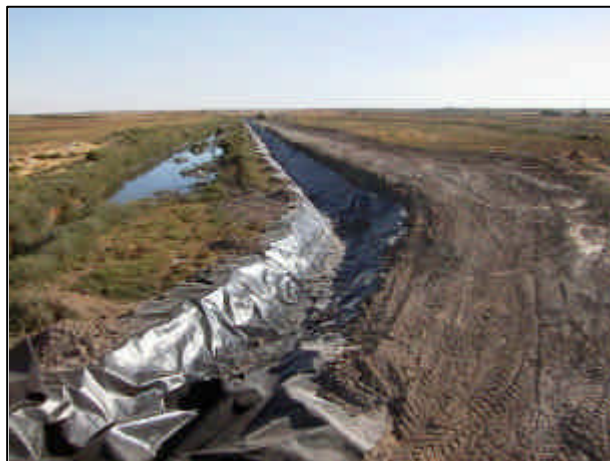
Filtering channel in Villacañas in the waterproofing process
